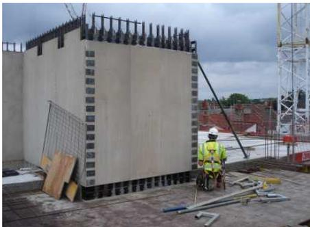
Flexibility to position walls ahead of slab (delay recovery)
