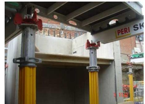
PSF interfaces with all leading proprietary deck / slab systems
