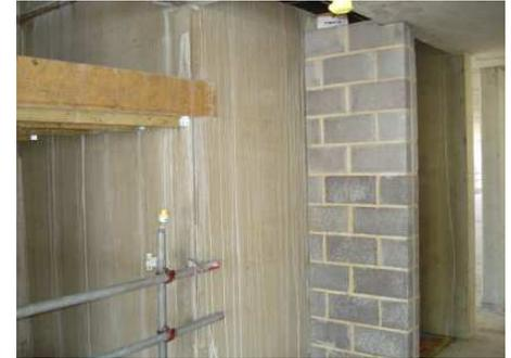
Blockwork and other finishes seamlessly integrate with PSF
