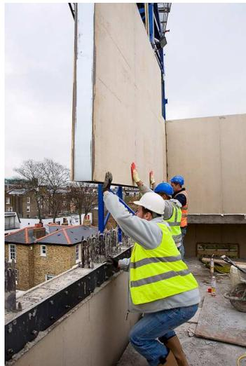
Small labour team required to construct 9 m long PSF wall
