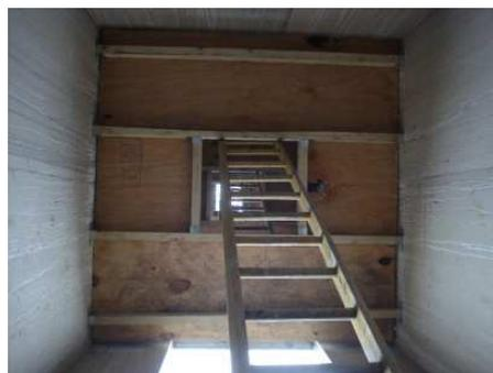
Safe internal access via hatches – removes need for scaffolding or external access tower in lift shafts
