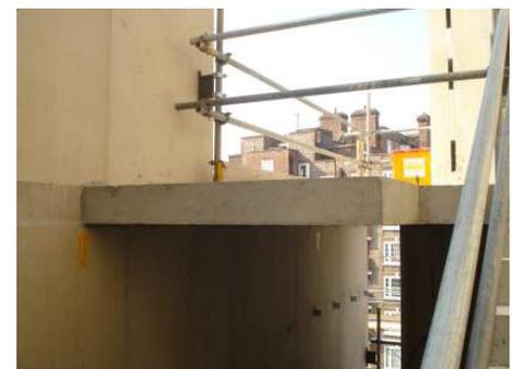
Verteka continuity strip allows cantilevered slab attachment
