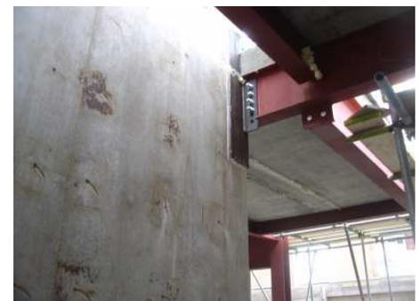
Steel frame can be directly attached to PSF walls
